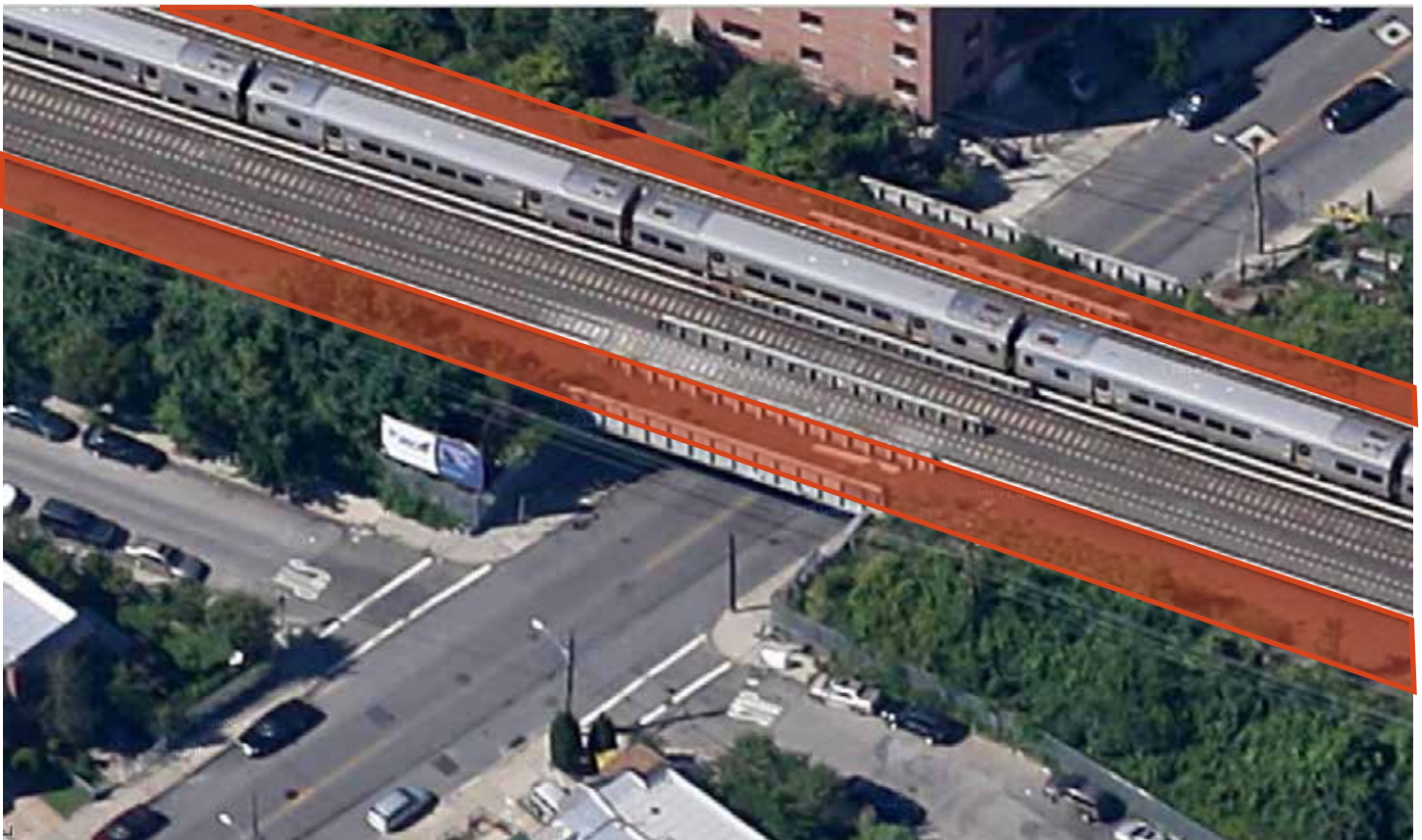
Above: Google map image of LIRR Main Line grade crossing at 57th Avenue and 85th Street in Elmhurst, Queens. The existing right-of-way has land for a potential expansion.
