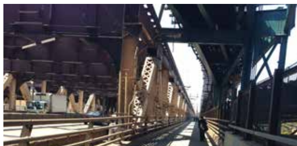
Edward Koch Queensboro Bridge Shared Pedestrian/Bicycle Lane
