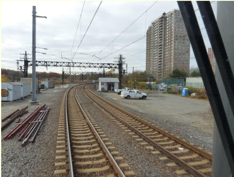
Co-op City, The Bronx, on the Hell Gate Route
