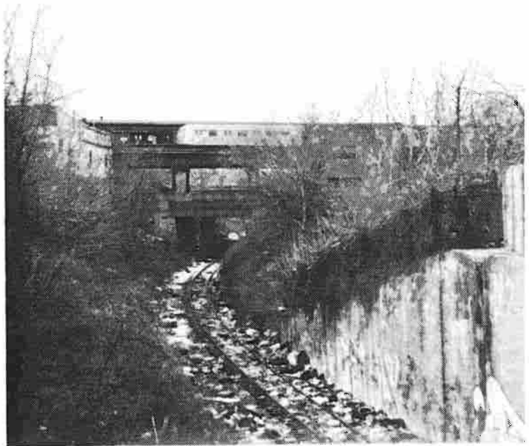
View looking west towards New Utrecht Ave. from 15th Ave.
