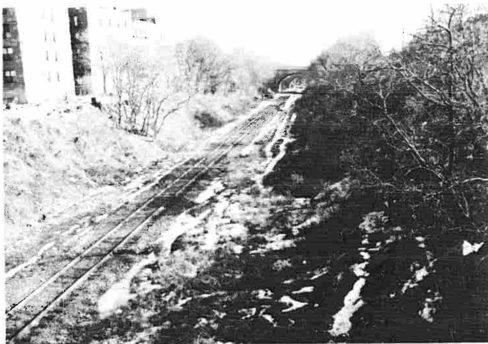
Looking south from 41st Ave. in Queens. Bridges in the background are, front to back: Woodside Ave., 43rd Ave. and 44th Ave. See page 17.
