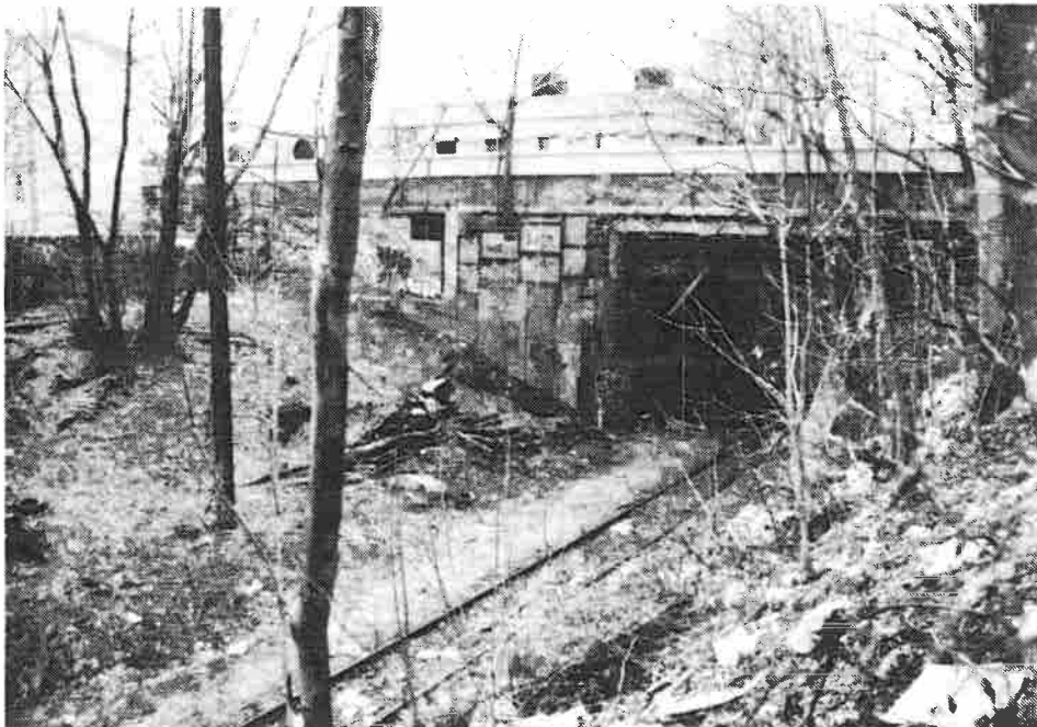
Looking south from East 16th St. towards the D train overpass, with the MTA substation behind it.
